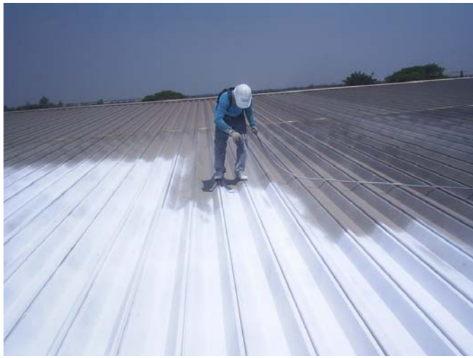
Max-kool coating by airless spray machine
