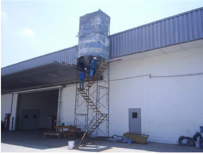
Scaffold set up
