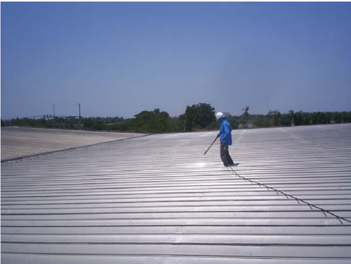
Cleaning & primer coating
